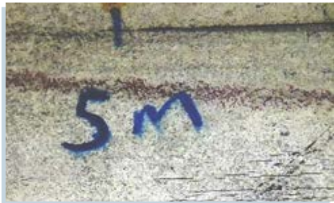
Pipe corroded by H 2 S
