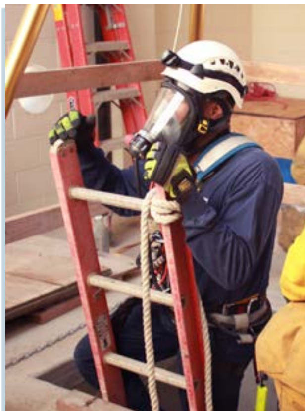
Worker entering a confined space
