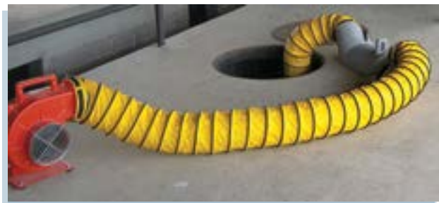
Always ventilate before beginning work
